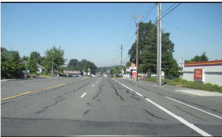
Power Prior to micro surfacing treatment
