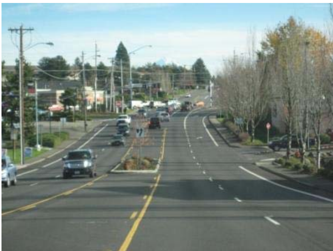
SE Powell Blvd looking east, after micro surfacing
